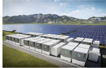
On-site solar + storage
