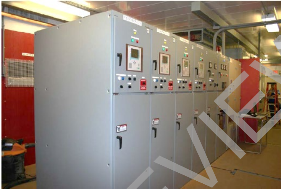
Figure 3.2 DC Switchgear Cubicle –courtesy DART
