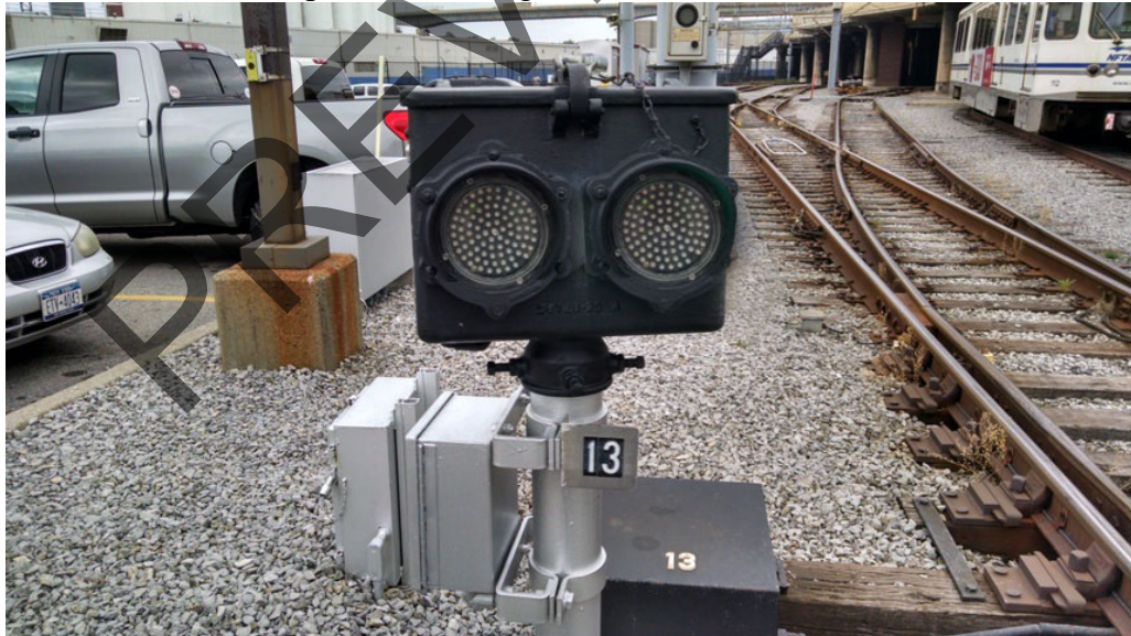
Figure 3.1 Dark Wayside Signal – Courtesy NFTA (modified by consortium)
