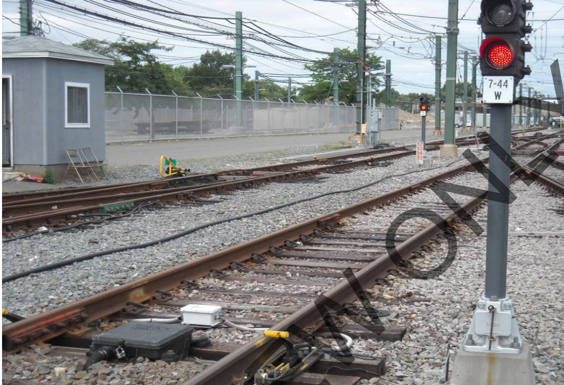
Figure 3.2 Stop Signal on a Wayside Signal
