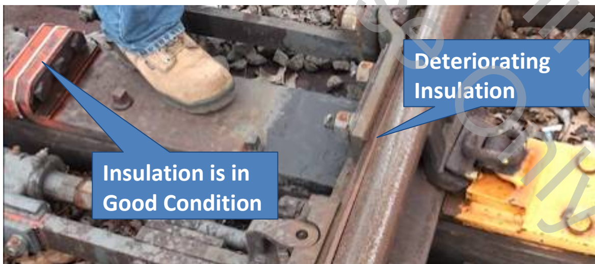
Figure 3.2 Insulation - Courtesy LIRR
