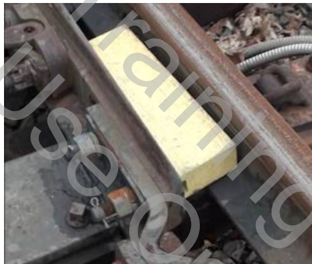
Figure 1.7 Block Wedged Tightly between Open Point and Stock Rail
