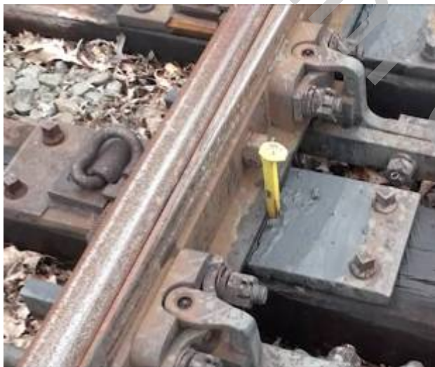
Figure 1.6 Spike Against Closed Point
