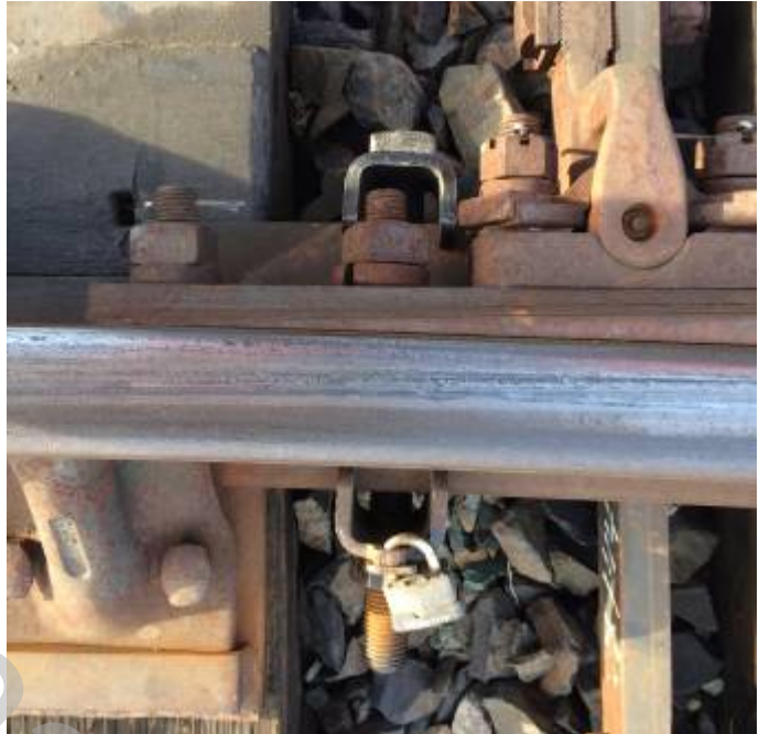
Figure 1.5 Switch Clamp in Use
