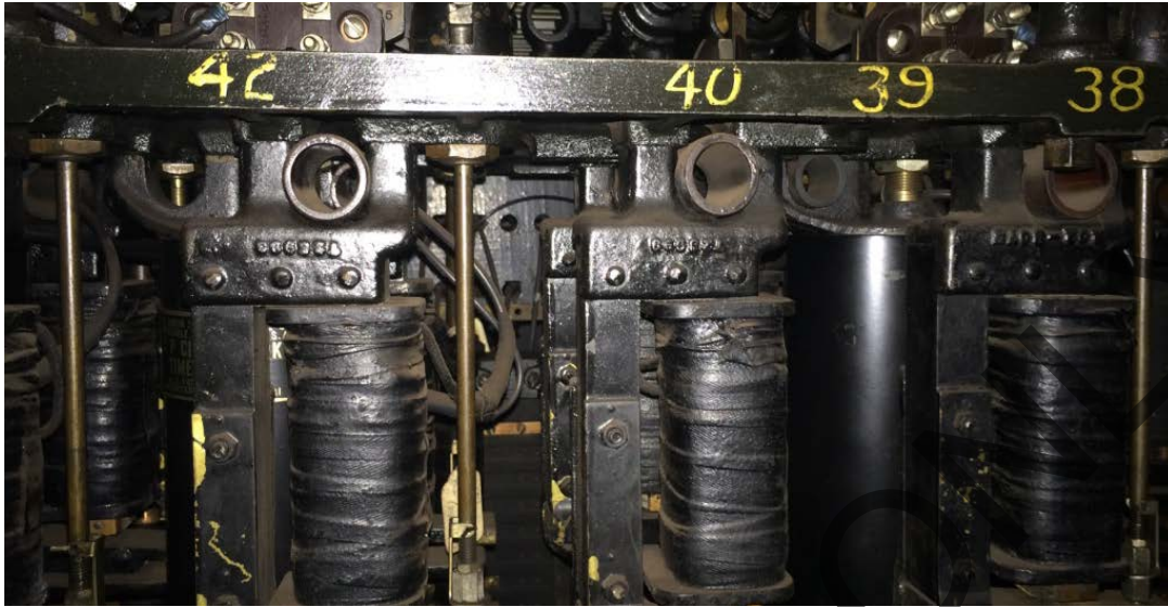
Figure 4 Magnets located in the rear of the lever machine
