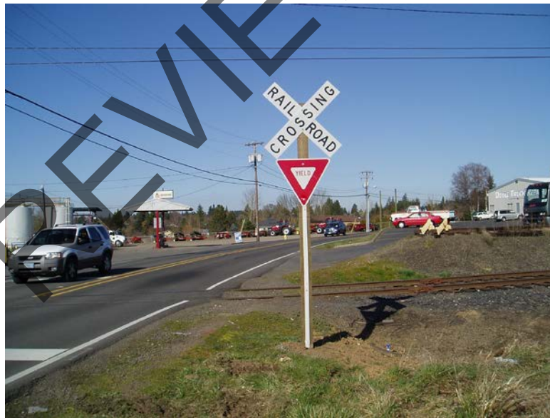
Figure 5 Passive highway grade crossing with a crossbuck mounted on an mast and with optional yield sign, Courtesy Oregon.gov
