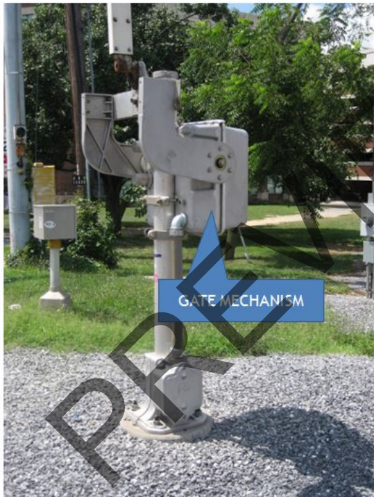
Figure 17 Gate Mechanism at a Highway Grade Crossing
