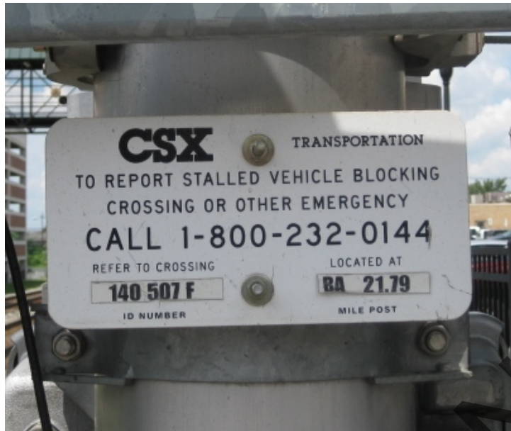
Figure 4 Highway Grade Crossing Sign Indication Crossing Identification Number and Phone Number for Emergencies – MDysart 2013
