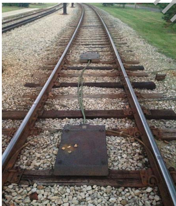
Figure 101.20 Impedance Bonds – Courtesy GCRTA
