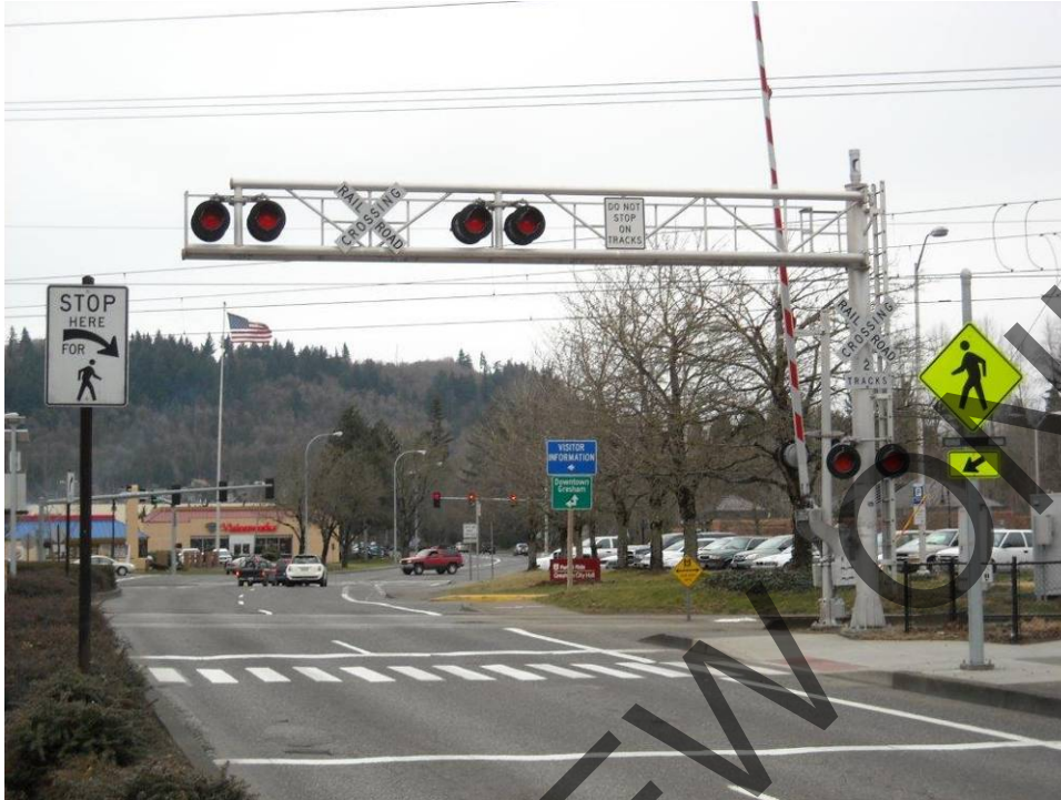
Figure 3.1 Clearly Visible and Maintained Signage at a Highway Grade Crossing
