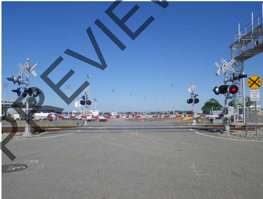
Figure 16 Four Quadrant Gate System with Both Entrance Gates Lowered and Exit Gates Lowered Creating a Sealed Corridor
