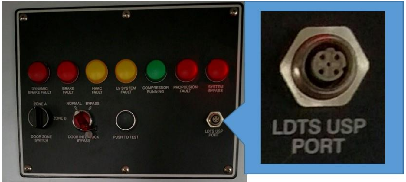
Figure 3.24 PTU Port on the FIP. Courtesy of PATCO
