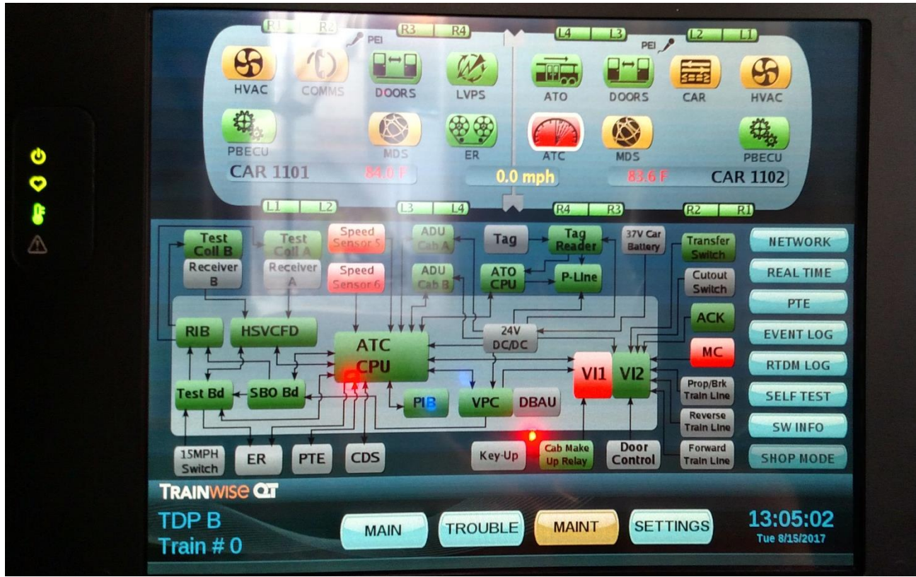
Figure 3.23 Train Display Panel on Maintenance Screen. Courtesy of PATCO
