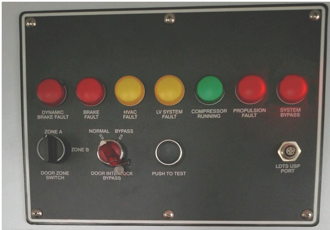
Figure 3.19 Fault Indicator Panel. Courtesy of PATCO
