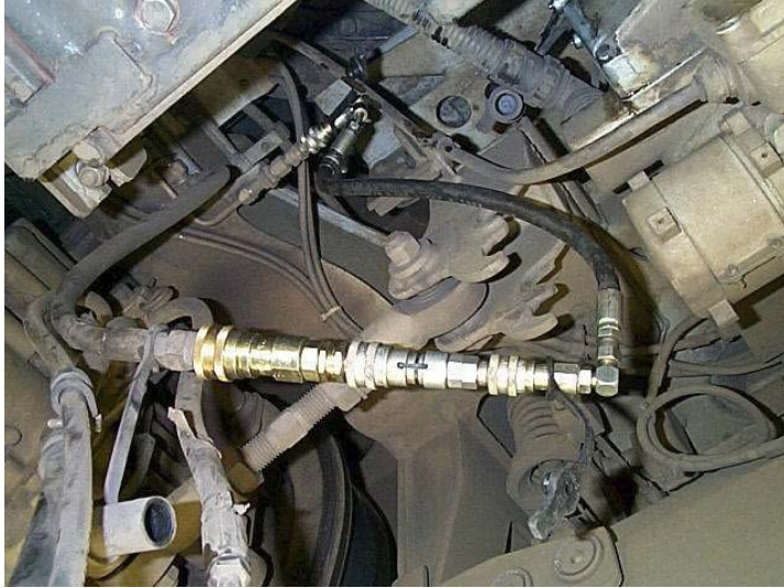
Figure 3.7 Flush Unit Connected to LRV –courtesy Denver RTD
