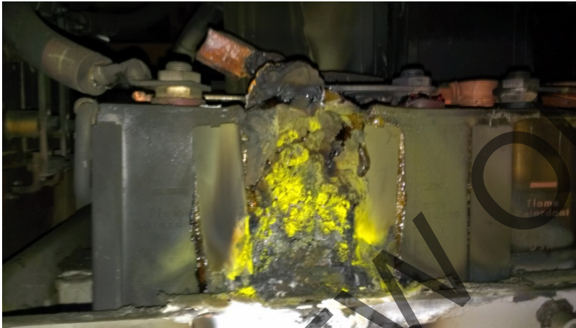
Figure 3.1 Leaking Battery Cell –courtesy BART
