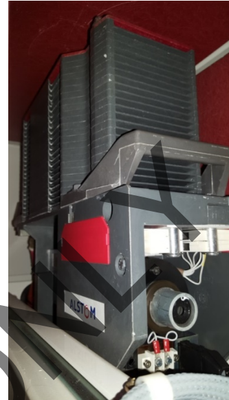
Figure 2.5 Side view of a High Speed Circuit Breaker –courtesy PATCO
