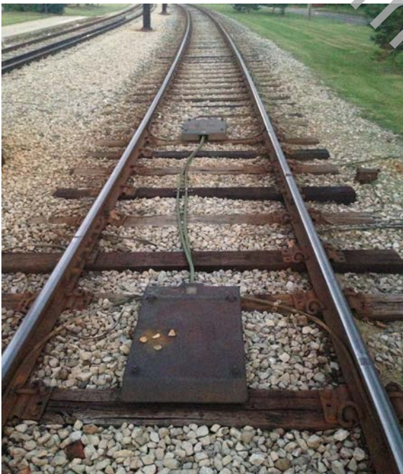
Figure 101.20 Impedance Bonds – Courtesy GCRTA
