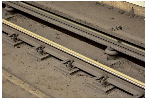
Figure 7 Third Rail system
