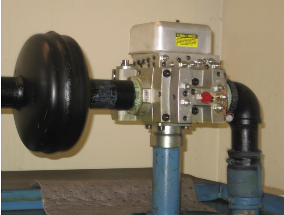
Figure 2.5 Small Muffler Used in Down Regulated Systems –Courtesy NYCT
