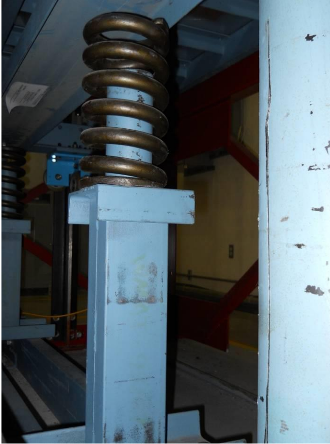
Figure 1.14 Spring Buffer –Courtesy WMATA
