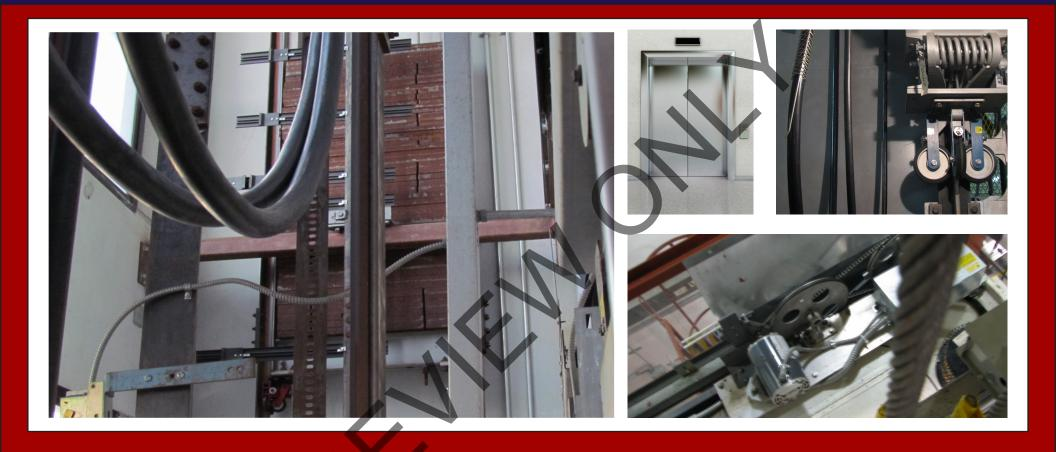
217: Elevator: Traction Elevator
