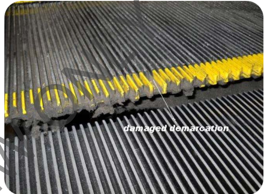
Figure 1: Damaged Demarcation
