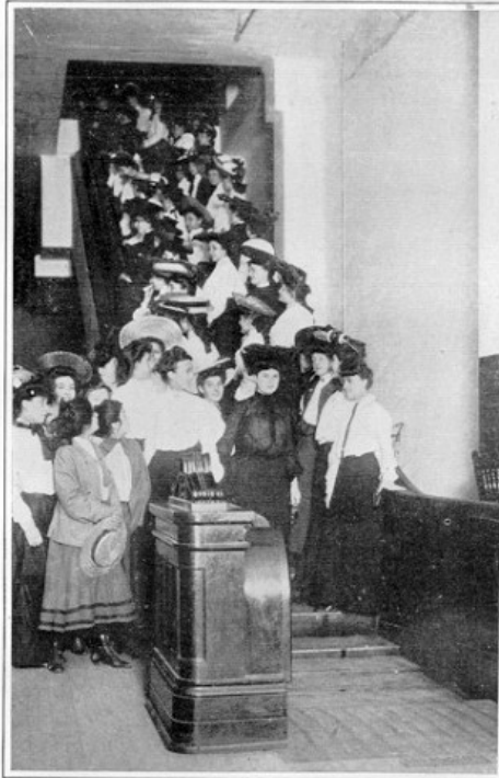
ELECTRIC TRAVELING STAIRWAY IN A DEPARTMENT STORE An escalator, operated by an electric motor, in a department store. Moving stairways, such as this, consist of endless belts, upon which one may stand or walk and be carried upward.
